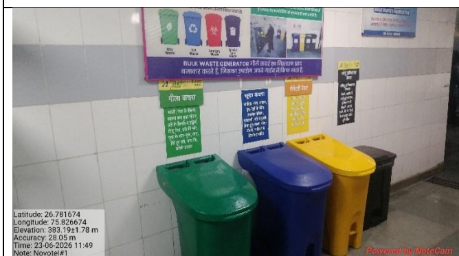
4 bin system at Hotel Novotel
